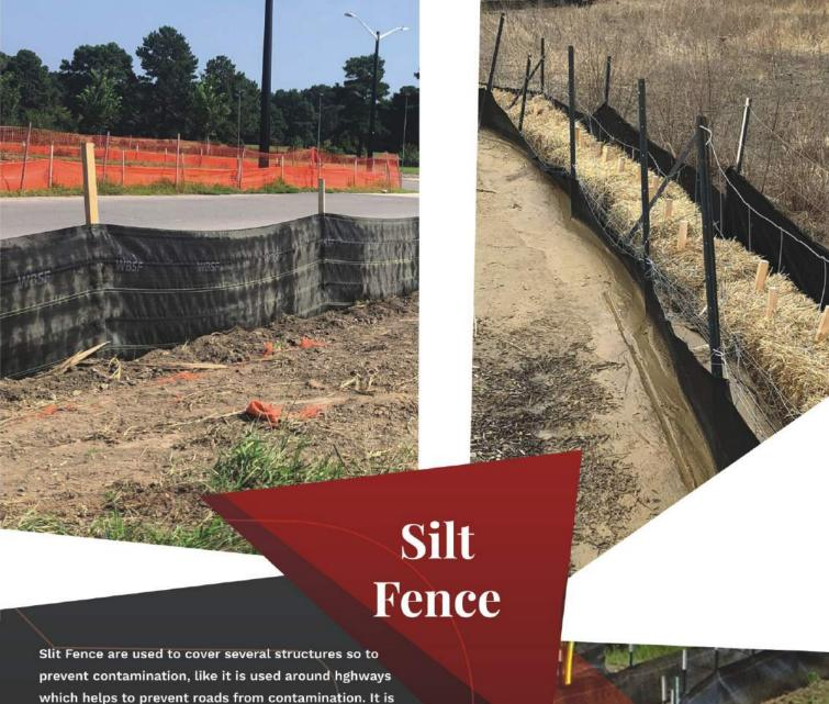
Slit Fence are used to cover several structures so to prevent contamination, like it is used around highways which helps to prevent roads from contamination. It is also built around water bodies to prevent soil erosion. The fences are made from woven fabric and offer high strength and a controlled level of water permeability.
